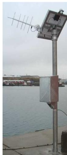
**Figure 2.** Econet Data Acquisition System.
